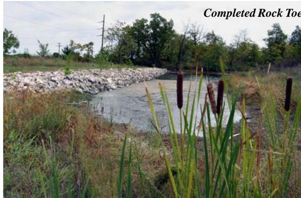
The project eliminated a total of 2095 feet of dangerous highwall which was from 15-20 feet away from the roads. There was a 15 foot drop over the highwall to the surface of the strip pit impoundment where the water depth ranged from 15-20 feet. Adding to the problem, the impoundment drained and seeped in an uncontrolled fashion saturating the roadbed, and creating flood and maintenance problems.
