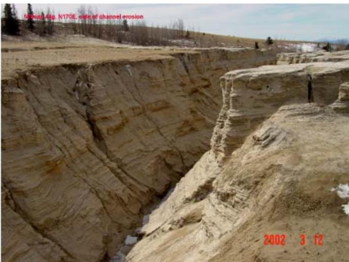
*Before — Channel erosion in fine grained mill tailings, approximately 50 feet deep with near-vertical side walls, looking northwest*
